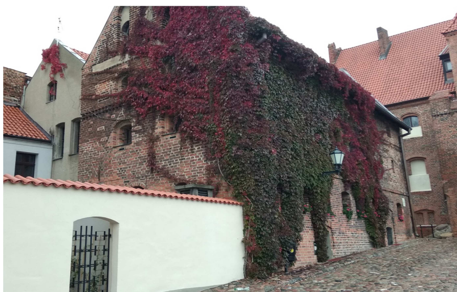
Fig. 1. A building at Podmurna Street in Toruń overgrown with a vine as an example of a vertical garden, Source: Katarzyna Ziemkiewicz, 2019
