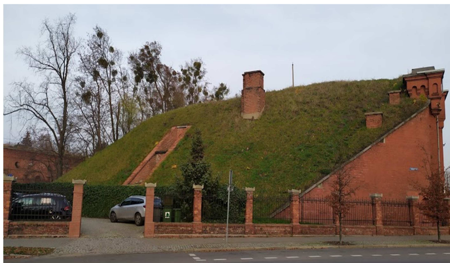
Fig. 2. Green roof on a fortress at Dąbrowskiego Street in Toruń Source: Katarzyna Ziemkiewicz, 2019
